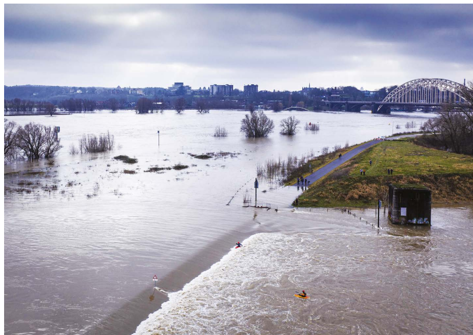
Flood waters breach a weir on the River Waal in the Netherlands in February 2021.
